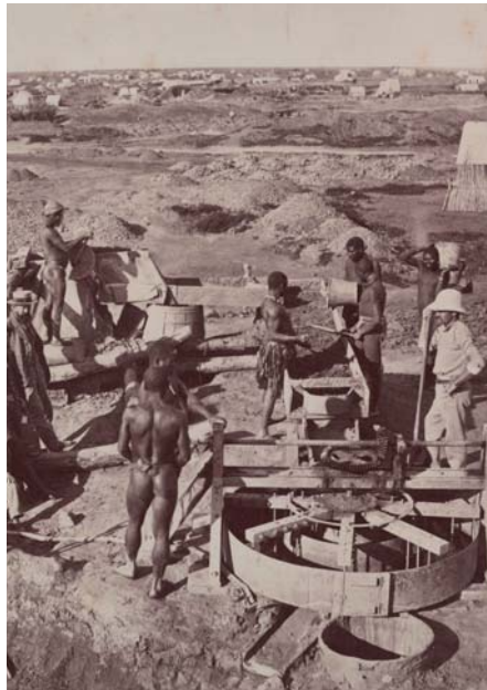
AVQ-A-004182-0046 Work in a diamond mine in South Africa, 1883
